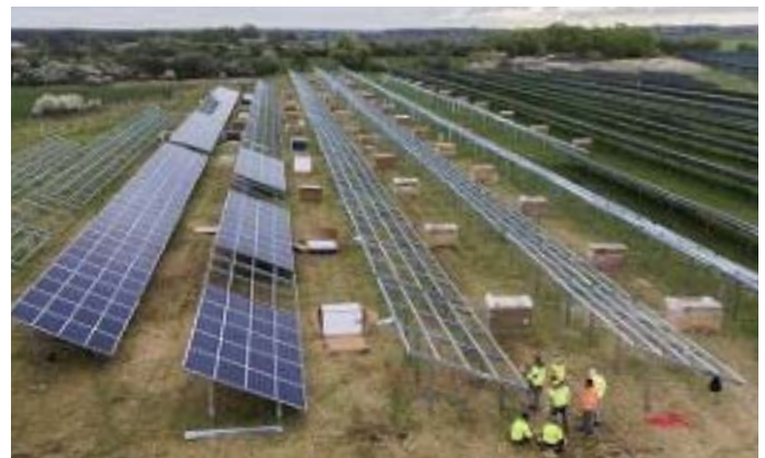
Digging of cable trenches and the relevant foundation work for the transformer stations.
